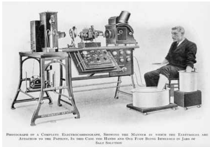
Figure 9: Electrocardiograph constructed by William Einthoven
